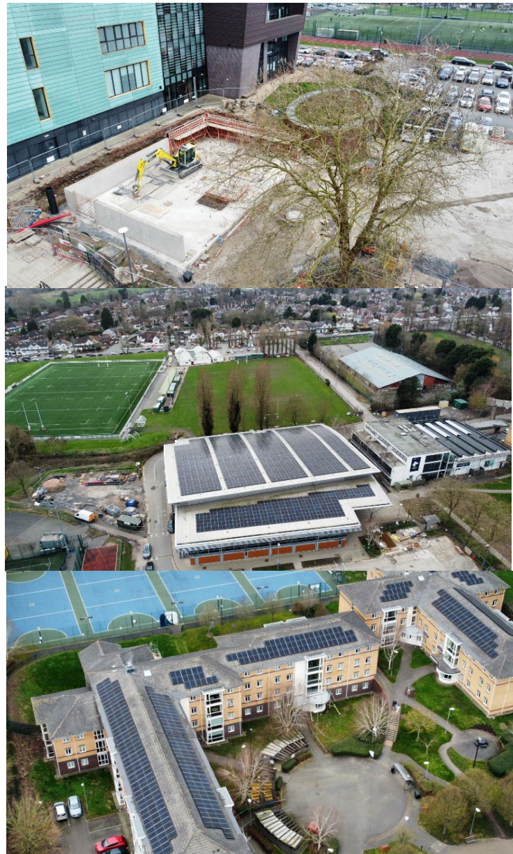
Drone footage taken at the Walsall Campus in February.
