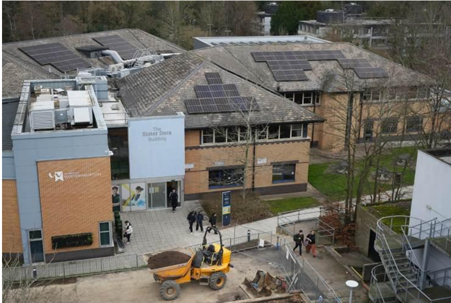
Image 1: Solar panels on the Sister Dora building and other buildings will significantly reduce the campus' carbon footprint.
